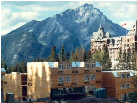
Construction of the quarters
